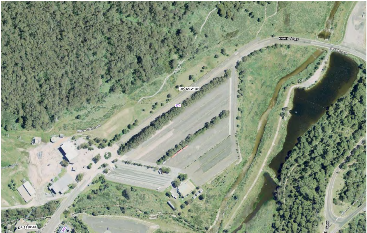
Figure 4: Aerial view of the subject site
